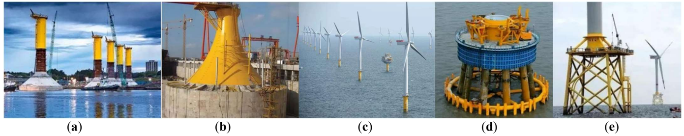
Figure 3. Common types of fixed-bottom offshore wind power foundations. (a) Blyth, UK; (b) Three gorges Xiangshui, China; (c) London Array, UK; (d) Donghai Bridge, China; (e) Alpha Ventus, Germany.
