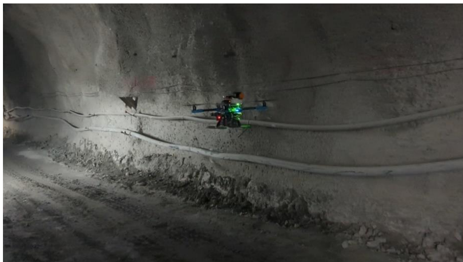
Figure 16. The drone moving along the tunnel in a low-light spot.
