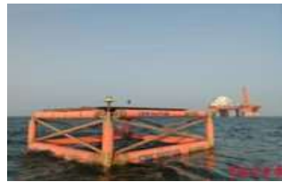
Figure 26. Global First Bamboo-Based Composite FPV Platform.
