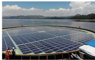
Figure 20. Magat FPV Project in Philippines.
