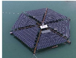
Figure 4. Hexagonal Tensioned Floating Island FPV Platform in Tianjin, China.
