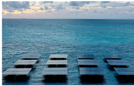
Figure 17. Solar Sea offshore FPV system.
