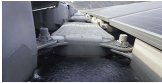
Figure 9. Pontoons bolted connection.
